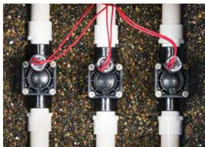
PGV-100G Valve Installed
