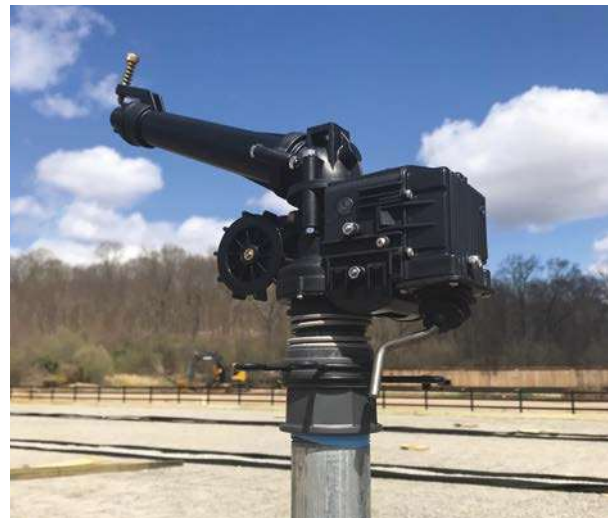
ST-1200-BR Rotor Installed
