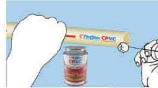
6. Solvent cement application
